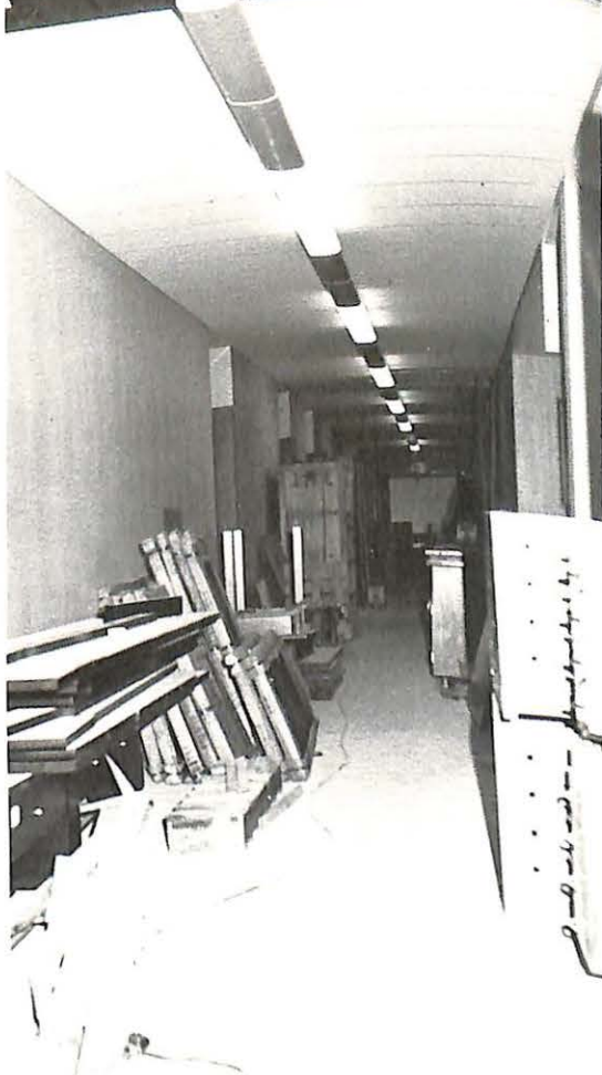
The interior of M. Earle Collins Science Hall nears completion.
